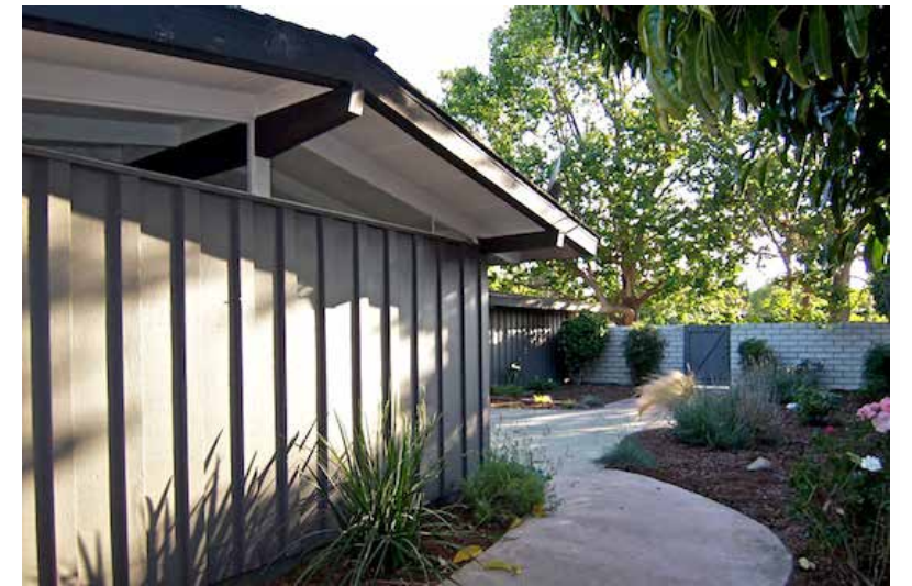
Sample Cement Fiber Board and Batten Installation
